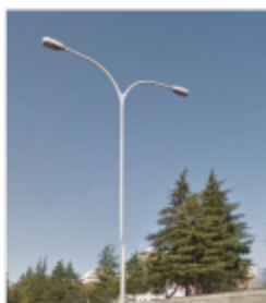
Typical WSDOT Angled Poles with LED Fixtures
