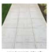
smooth concrete sidewalk
